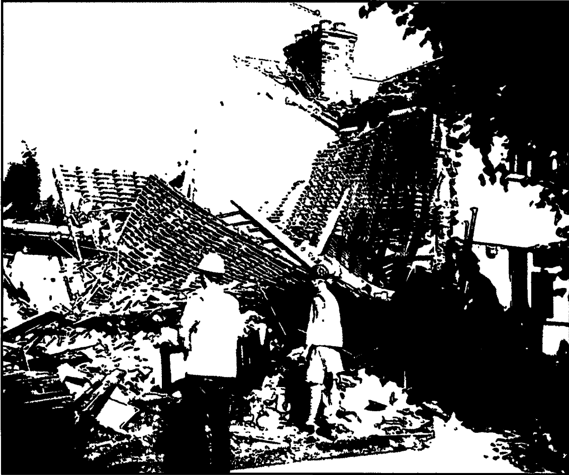
Figure 1 Aftermath of a gas explosion, following damage to an underground gas service pipe
