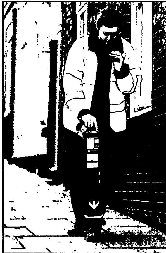
Figure 4 Using a cable locator
